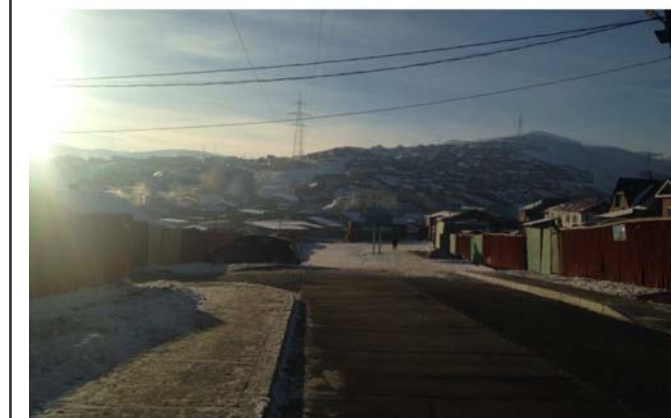
Improved road newar khoroo administration
